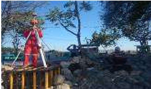
Figure 4: Determine Point Control.
